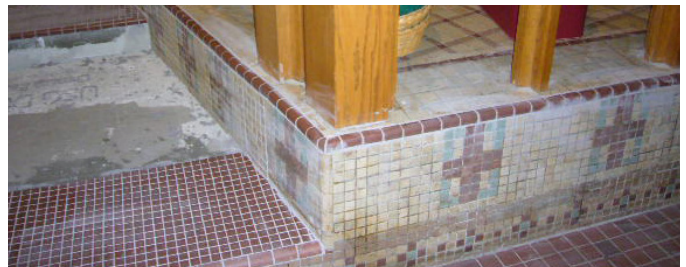
Tile work continued in the church this week. Photo: Jim Gremminger
